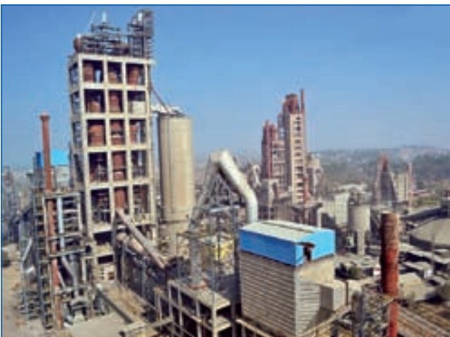
A view of new clinkerisation plant at Narsingarh
