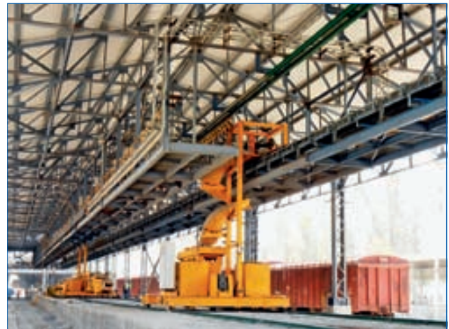
Cement loading facility at Imlai Plant
